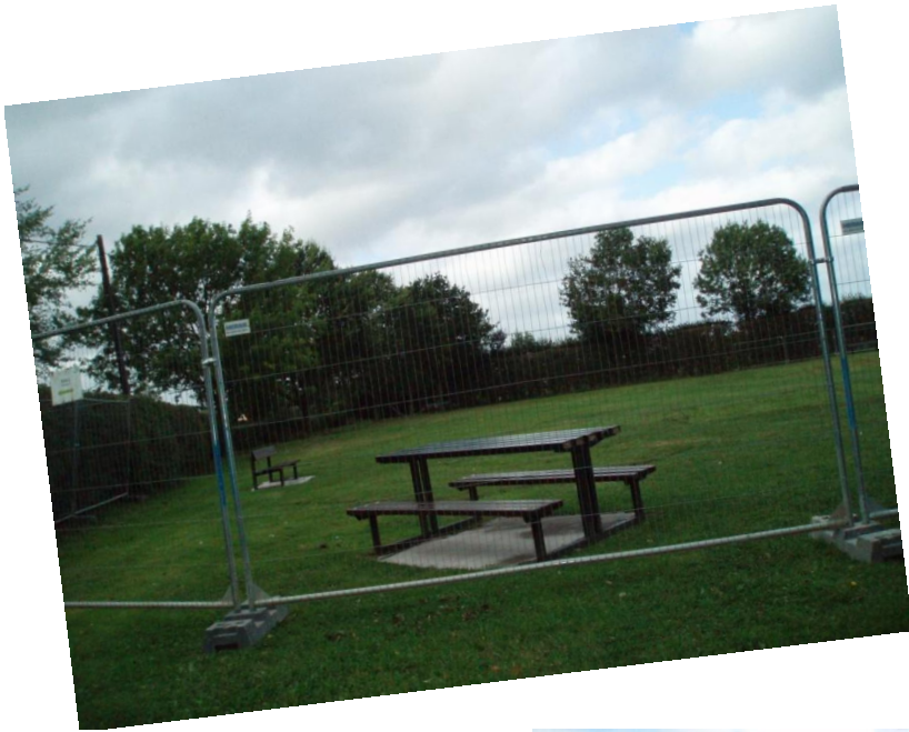
September 12 th – Fence and cabins in place
